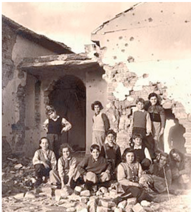
Destruction of childrens' house - Kibbutz Yad Mordechai 1948
